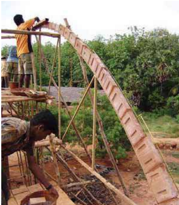
Figure 5: Precision being executed at site
